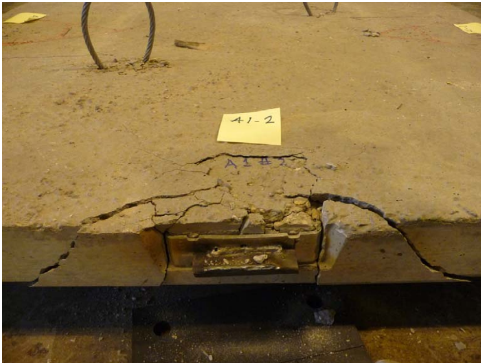
Figure 33 – Test A1-2 Failure Mode – top side view
