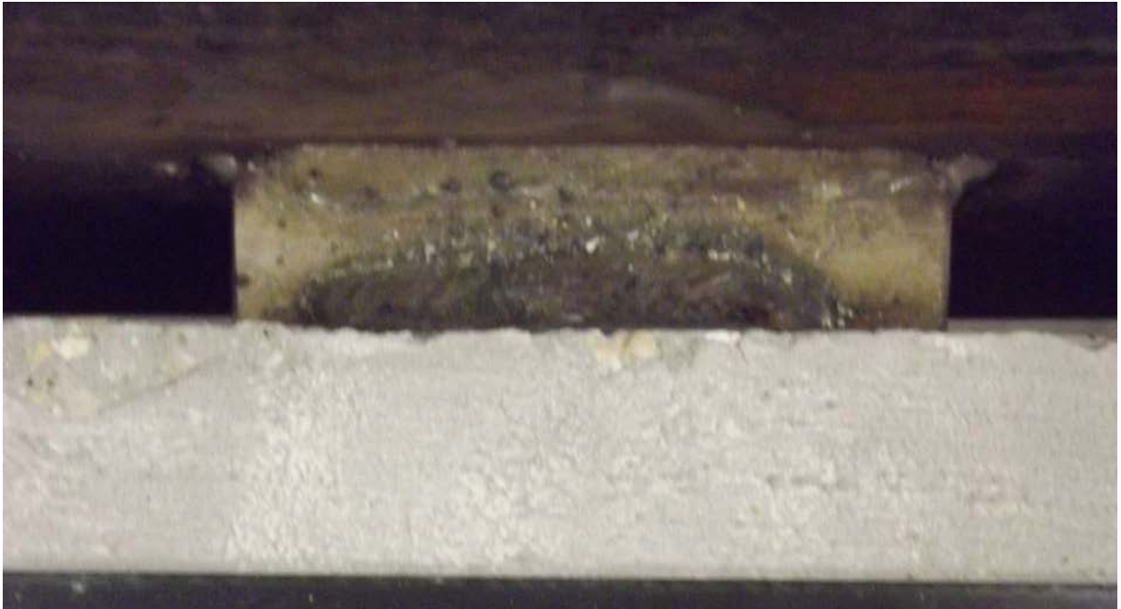
Welded Connection – Slug to VC4 faceplate and loading plate
