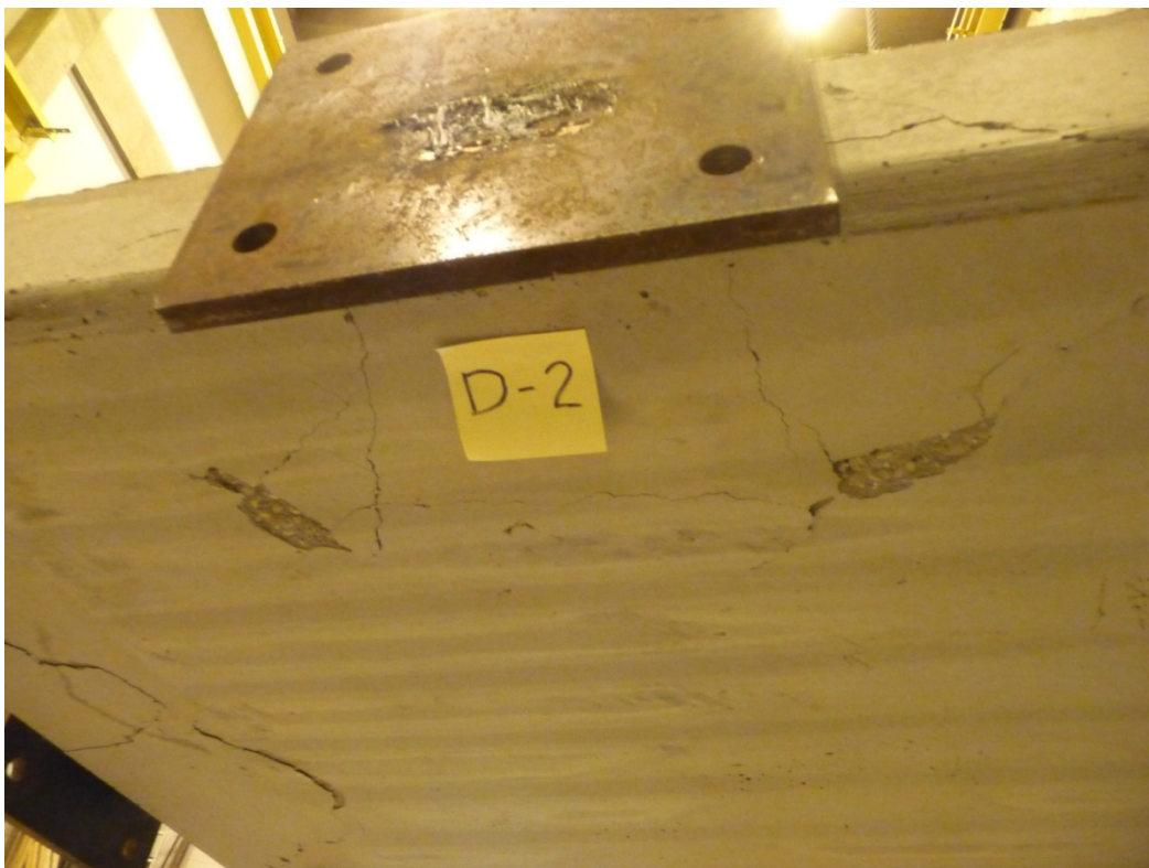
Figure 66 – Test D-2 Failure Mode – bottom side view
