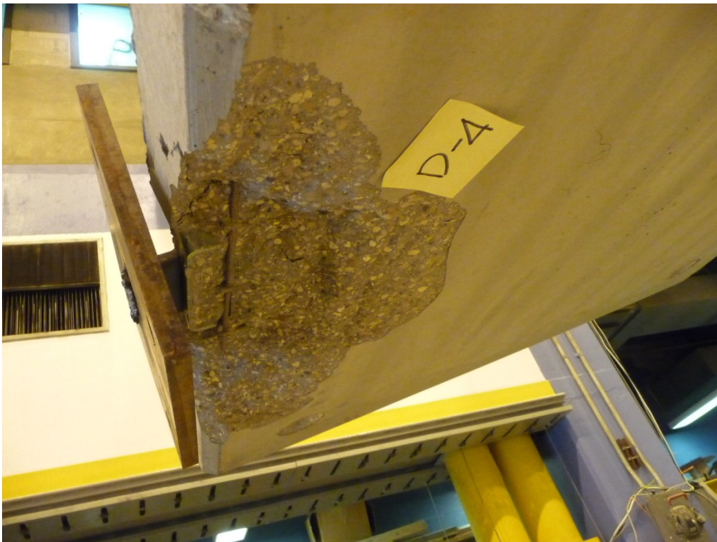
Figure 70 – Test D-4 Failure Mode – bottom side view
