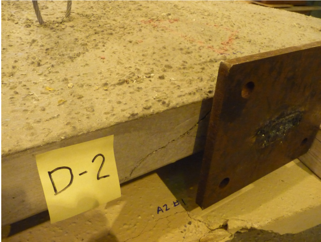
Figure 65 – Test D-2 Failure Mode – top side view
