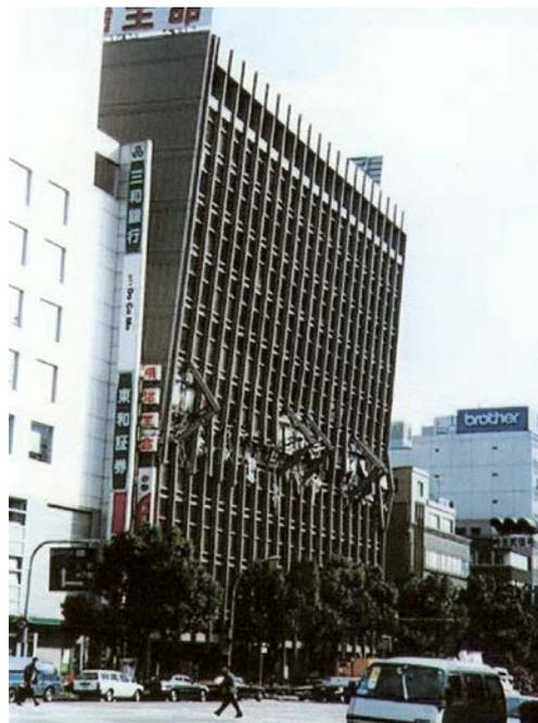
Figure 1c. Example of soft story collapse.
