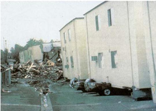
Figure 1a. Example of soft story collapse.
