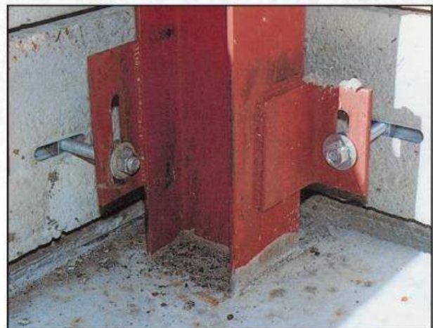
4-WAY ADJUSTMENT BOLTED TO FRAMEWORK.
