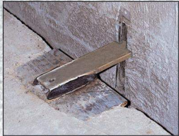
2-WAY ADJUSTMENT WELDED TO FRAMEWORK USING A NOTCHED STRAP.
