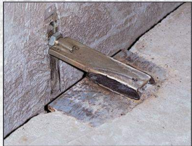
2-WAY ADJUSTMENT WELDED TO FRAMEWORK USING A THREADED STRAP.
