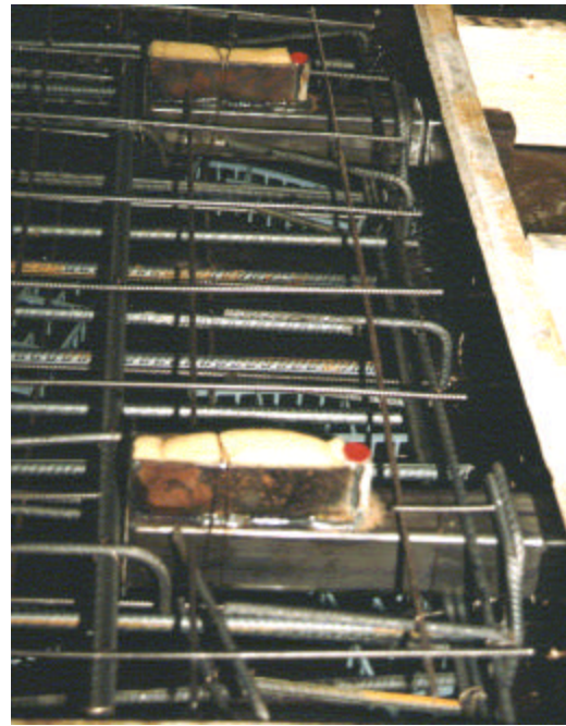
Picture 3. Reinforcement in the end with two units.
