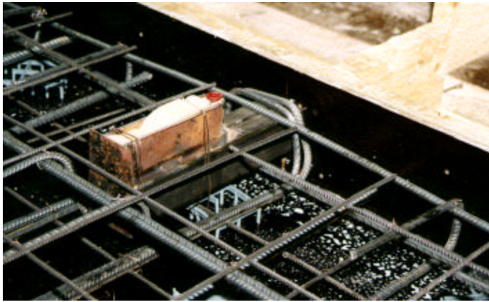
Picture 2. Reinforcement in the end with one unit.
