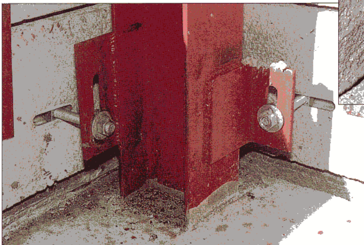
4-WAY ADJUSTMENT BOLTED TO FRAMEWORK.
