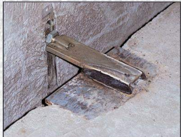
2-WAY ADJUSTMENT WELDED TO FRAMEWORK USING A THREADED STRAP.
