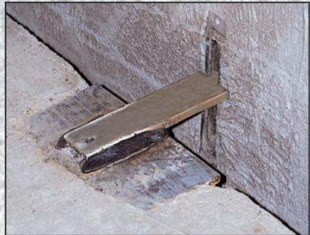
2-WAY ADJUSTMENT WELDED TO FRAMEWORK USING A NOTCHED STRAP.
