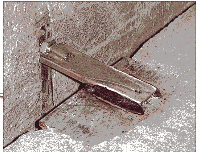
2-WAY ADJUSTMENT WELDED TO FRAMEWORK.
