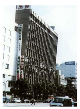
Figure 1c. Example of soft story collapse.
