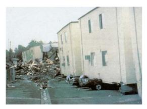
Figure 1a. Example of soft story collapse.
